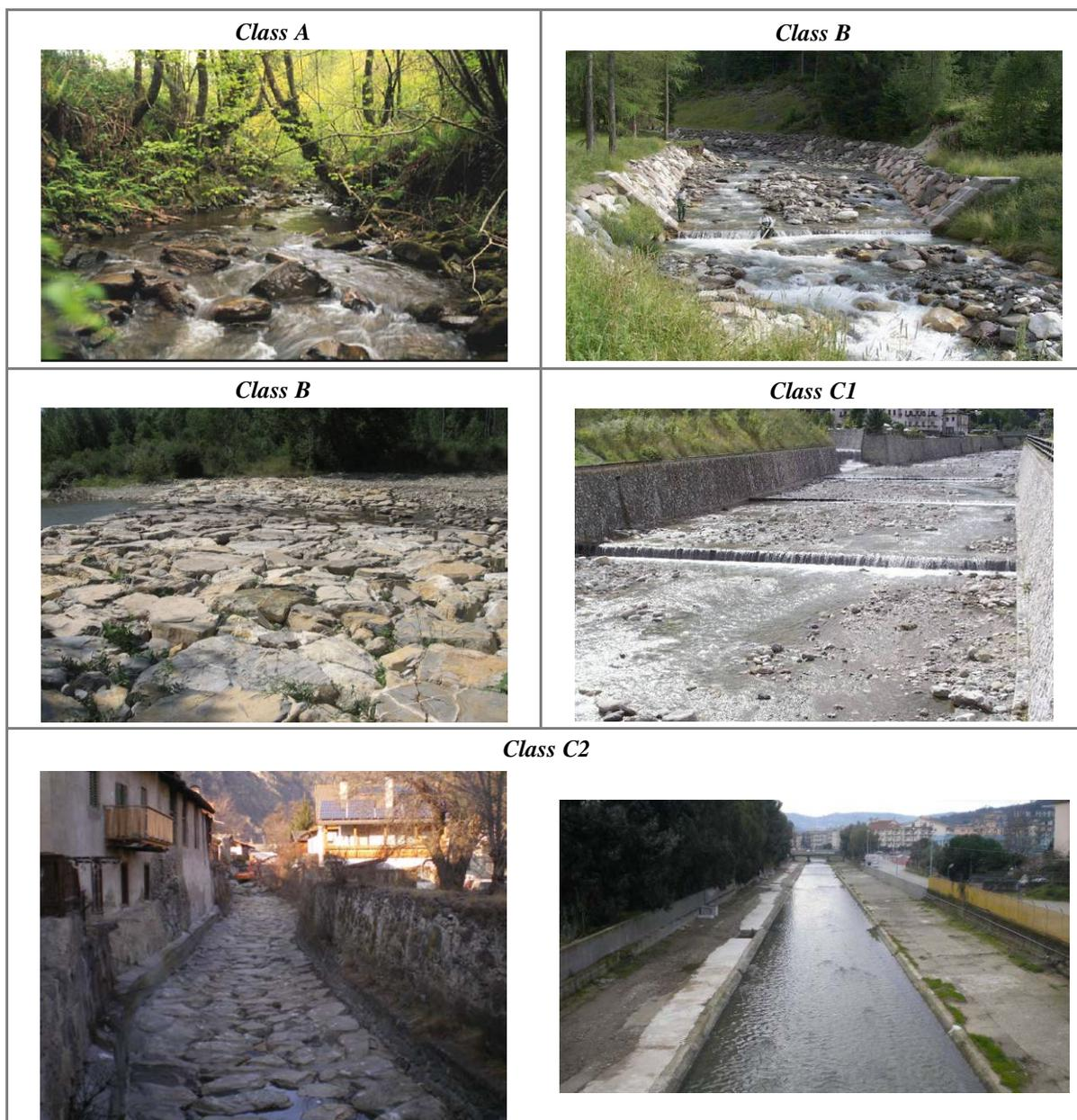
**Figure 73** – Other grade control structures and revetments. *Class A*: total absence of other grade control structures or revetments. *Class B*: presence of sills (first row on right) or mass ramps (second row on left) with low density. *Class C1*: various sills and partial bed revetment. *Class C2*: total bed revetment with impermeable systems. If such revetments occur along most of the reach (> 80%), an additional score of 12 is assigned.
