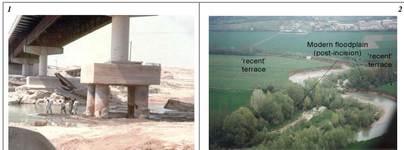
**Figure 81** – Field evidence of incision. (1) Exposed bridge piers. (2) Differences in level between modern (post – incision) floodplain and “recent” terrace (the latter corresponding to the pre – incision floodplain).
