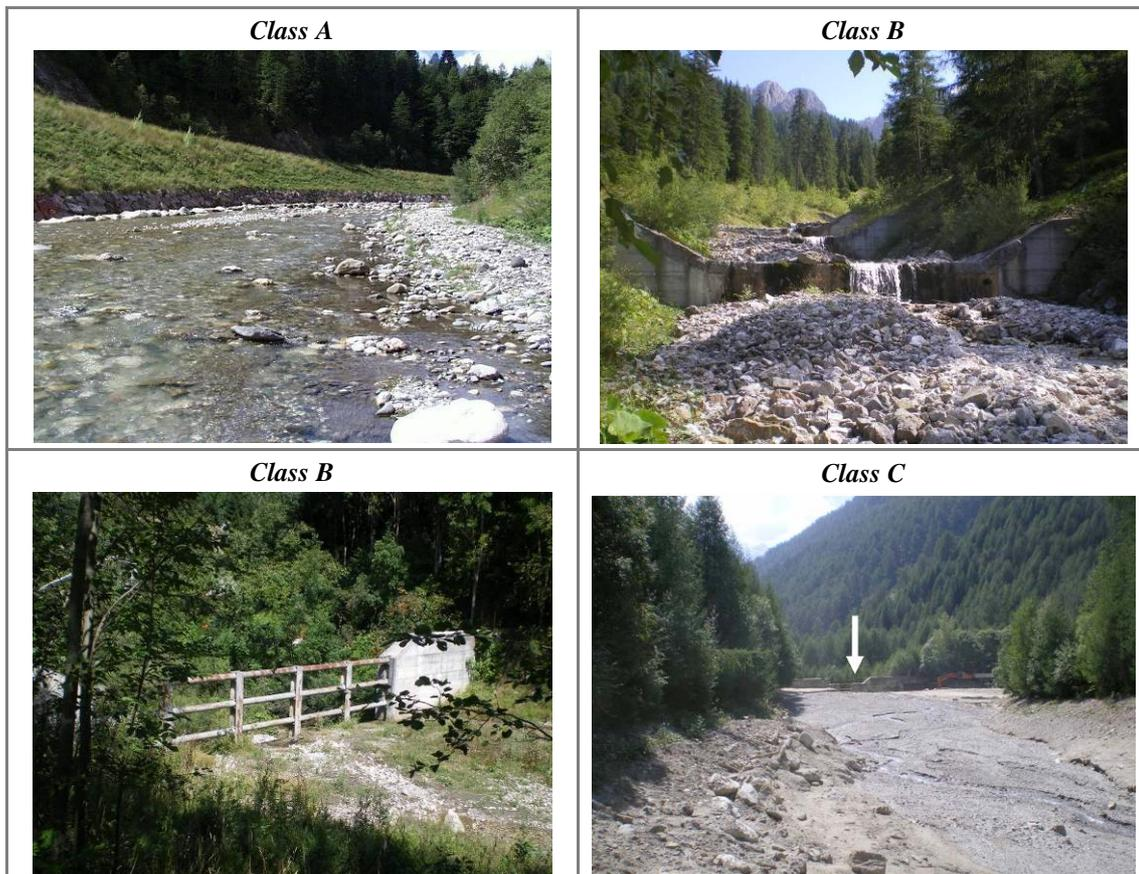
**Figure 20** – Longitudinal continuity in sediment and wood flux. *Class A*: absence of discontinuities. *Class B*: up on the right, filled consolidation check dams; low on the left, open check dam. *Class C*: a check dam (arrow) with total interception represents a complete alteration of longitudinal continuity in the reach downstream from the check dam.
