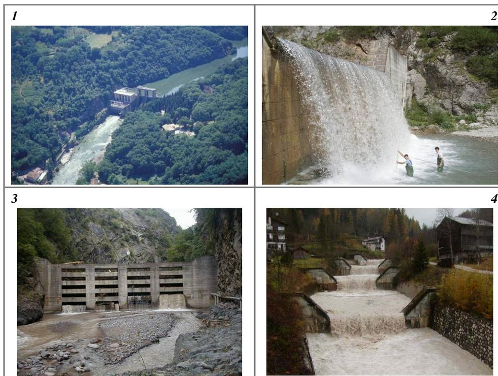
**Figure 55** – Transversal structures of alteration of sediment discharges in mountain areas. (1) Dam; (2) retention check dam; (3) open check dam; (4) sequence of stepped consolidation check dams.
